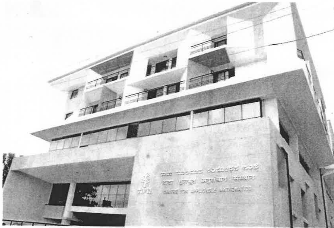
FOCUS ON APPLICATION: The building of the Tata Institute of Fundamental Research-Centre for Applicable Mathematics at Yelahanka New Town in Bangalore
